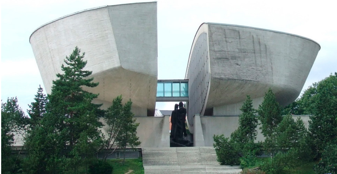
1. Museum of the Slovak National Uprising in Banská Bystrica, main building
