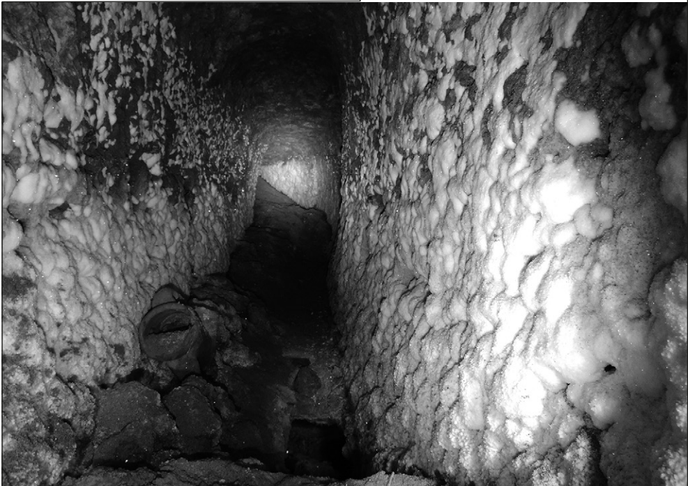
Fig. 8. Tunnel in the east wall of the inner chamber of the Hellenistic gate: top, view toward the back end where it turns to the northwest; thick salt efflorescence covers the walls; right, sunken part of the channel cut into the floor of the tunnel inside the chamber of the Hellenistic gate and covered with thin stone slabs (PCMA–University of Delaware Berenike Project/photos M. Woźniak)
