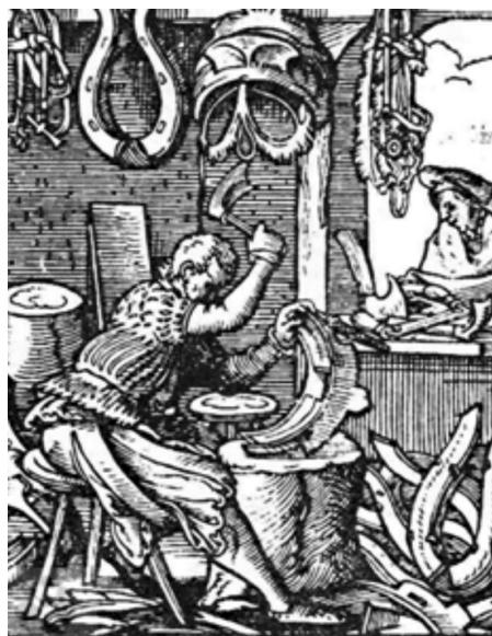
Figure 2. Work of saddlers 5
