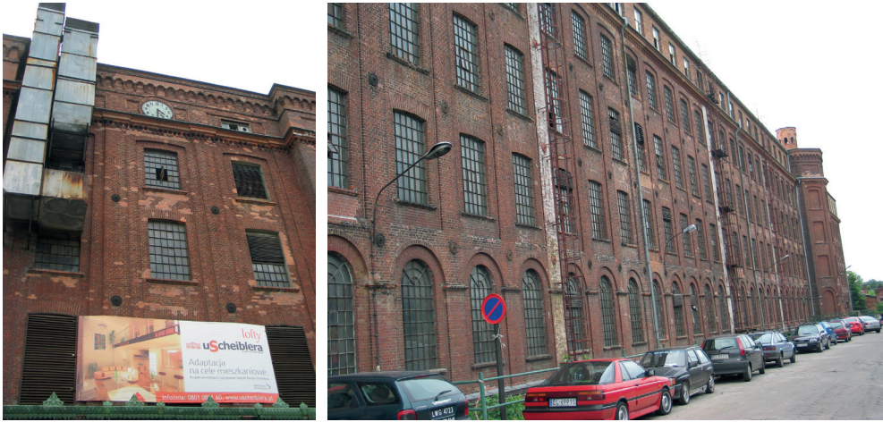
Figs 5–6. The historic spinning plant before adaptation for lofts (2006)
