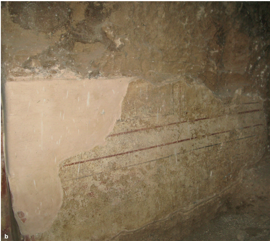
2a. Imitation of a built intrados in the arcosolia of rock-cut T.23; b. imitation of marble panels on the wall of the dromos leading to the entrance of T.22 (Phot. V. Lysandrou).
