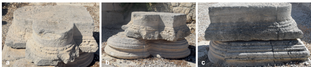
16a-c. Colonnaded hall: Attic half-bases (cat. no. 2) and Doric half-capitals (cat. no. 3) of the south-west heart-shaped pillar (Phot. P. Pensabene).
