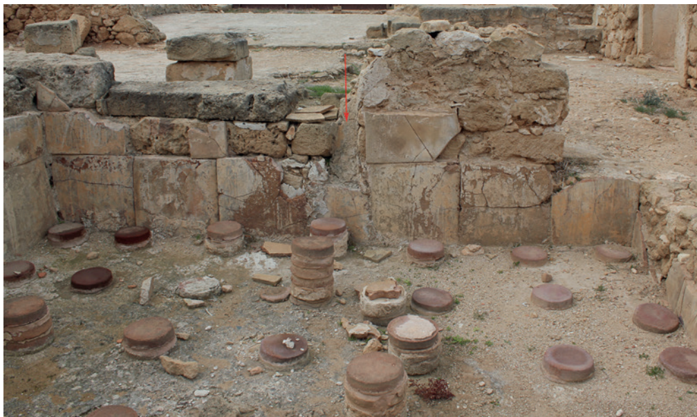
9. West wall in room R 17; the circular air duct can be seen in the middle (Phot. S. Christodoulou).
