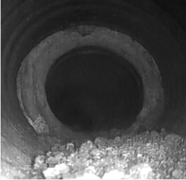
6. Fingerprints impressed in the inner mortar sealing of the joint between pipes; picture taken with an endoscope camera (Phot. M.M. Romaniuk).
