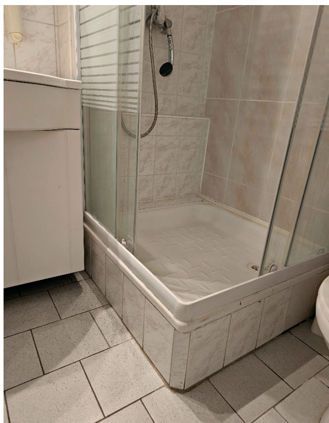
Figure 3. Shower tray – high threshold, no handles, no seat, no shelf for cosmetics
