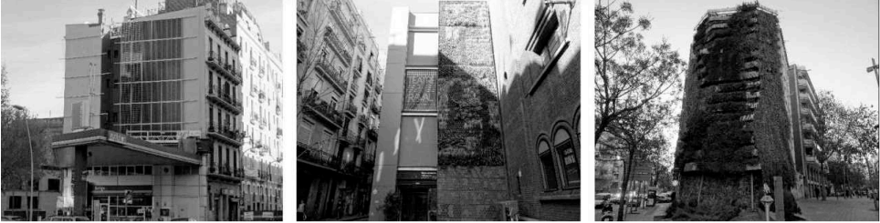
Fig. 28–30. An example of party-wall with solar panels and two other with vertical gardens. Source: Antoni Remesar, Bibiana Crespo-Martin.
