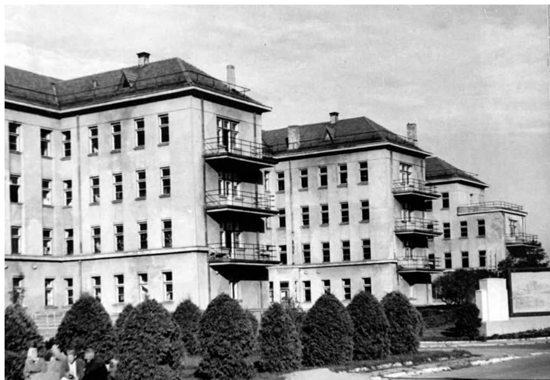
15. Vytautas Magnus University Clinics, architects Urbain Cassan, Elie Ouchanoff and Feliksas Bilinskis, part of the complex has been opened in 1939. Archive of KTU Institute of Architecture and Construction, album of Stanislovas Lukošius
