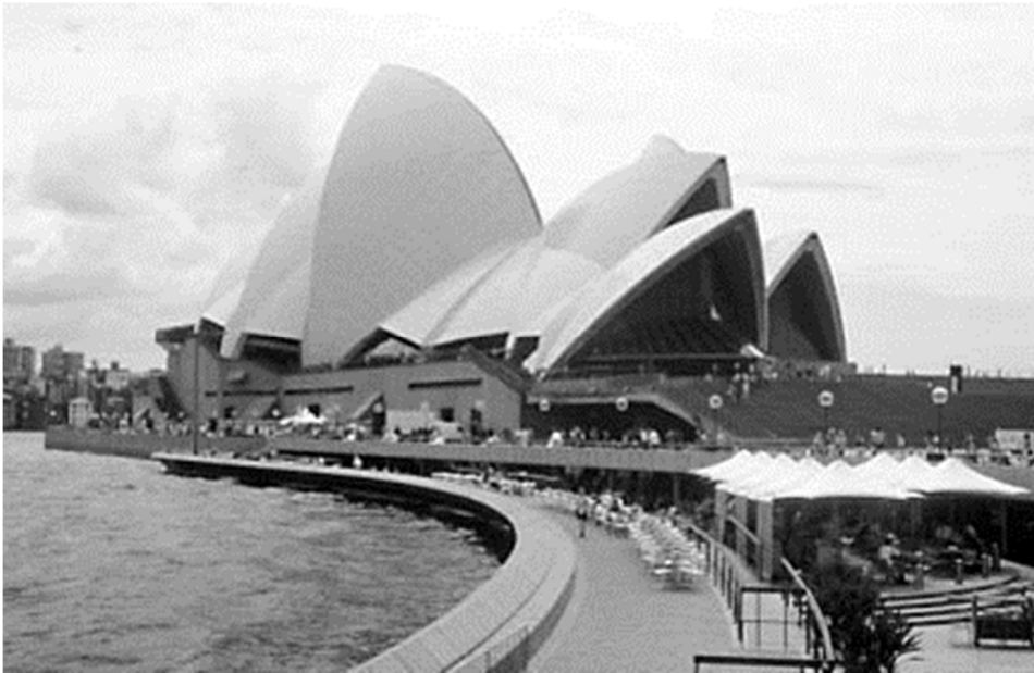
Figure 2. Exterior View of the Sydney Opera House.
