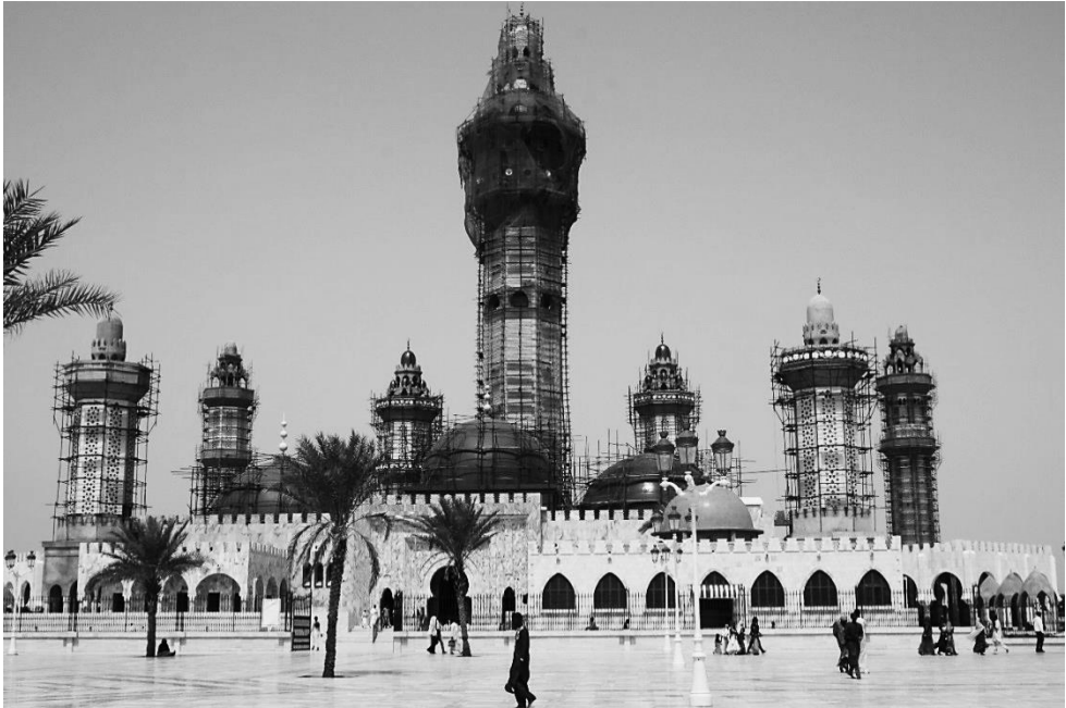
Great Mosque in Touba during renovation July 2015, photo B. NDiaye
