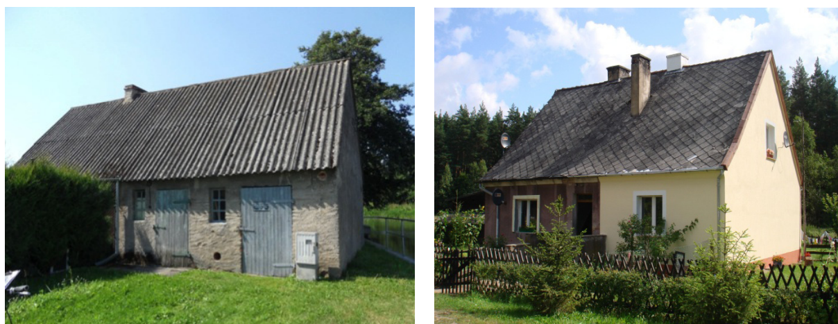
Figure 3. Asbestos-cement building roof covering A – corrugated asbestos cement sheets, B – flat asbestos cement sheets Author: Małgorzata Krówczyńska
