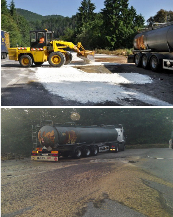
FIGURE 7 NEUTRALIZATION OF NITRIC ACID LEAK HYDRATED LIME
