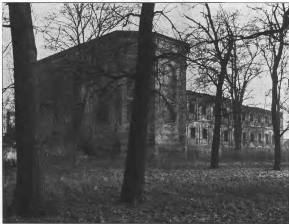
Illustration 2. The present-day condition of the estate; photo Pawel Warzynowski
